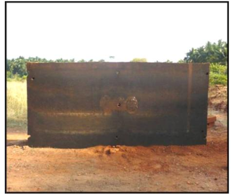
ATREE is building a new field station at Singampatti, in Tirunelveli district of Tamil Nadu. This eco-friendly structure is being built using rammed earth like the one seen in the picture.
