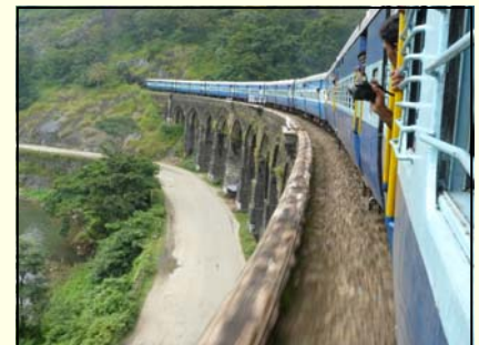
The spectacular Aryankavu viaduct Photo: T. Ganesh
